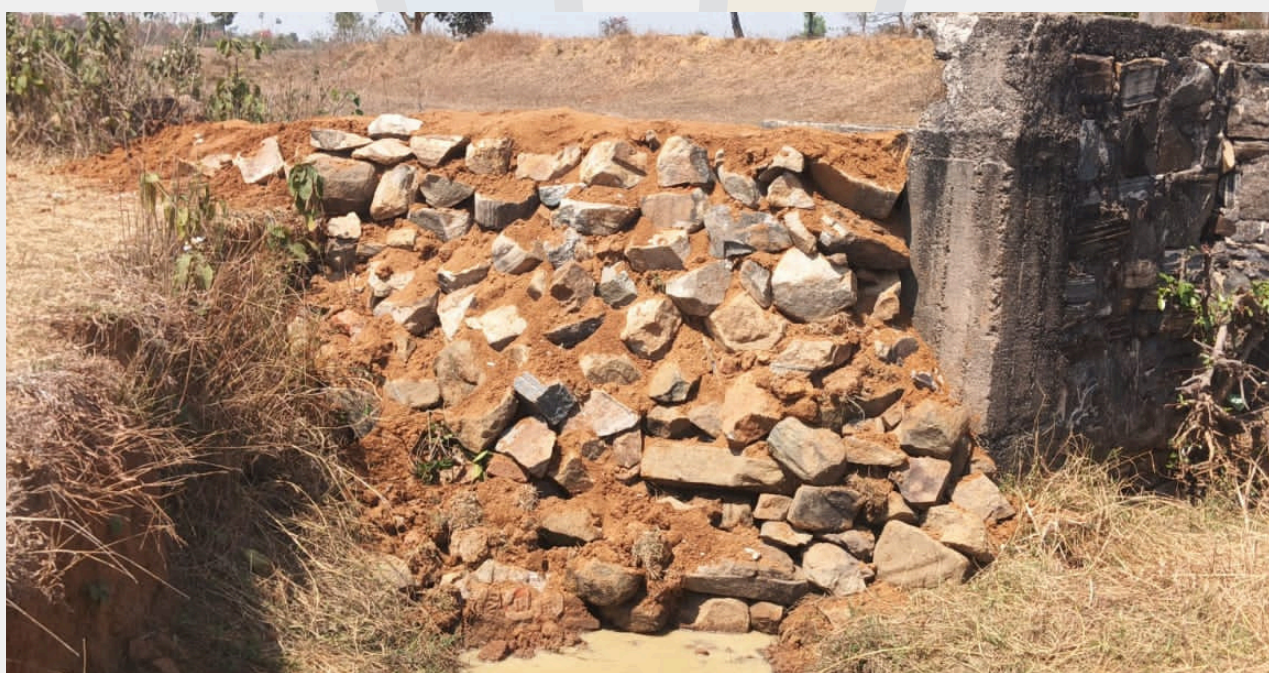
Guard wall after repairing
