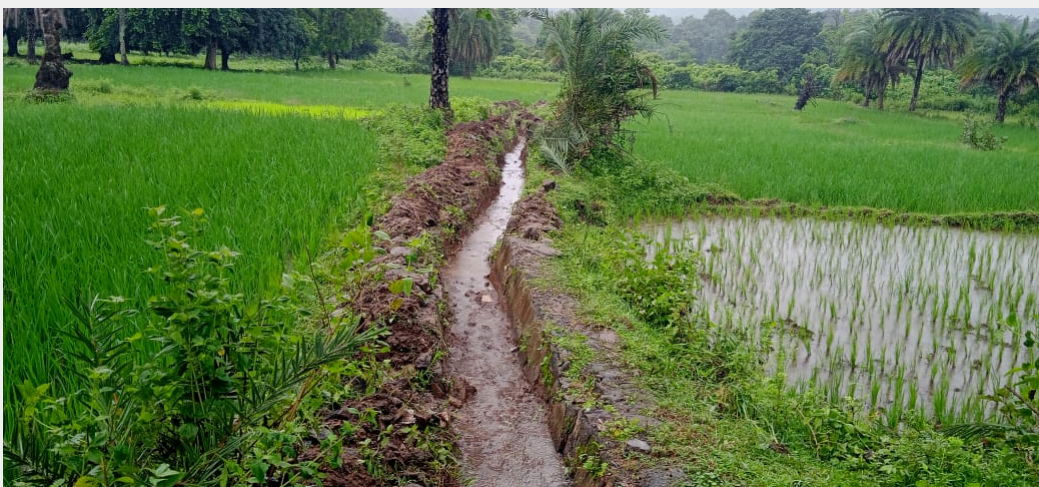
Farm land after building unpaved drain for irrigation
