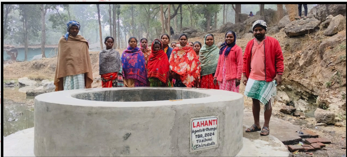
Water storage structure renovated to concrete well after intervention
